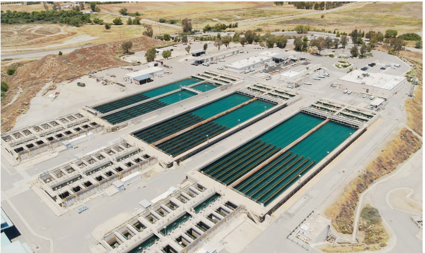
Aerial view of Robert A. Skinner Water Treatment Plant.
